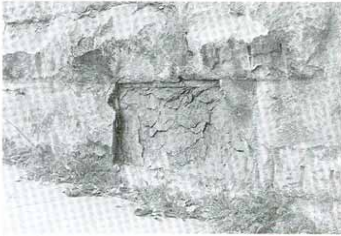
Typical sheeting in exfoliating limestone at the base course of a retaining wall (ca. 1880). The stone is sluffed off in thin layers. Compare to exfoliation in concrete shown in the following photograph.
